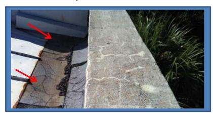
b. Clean existing coatings from metal roof and inspect thoroughly for holes that penetrate the metal. Wire brush or otherwise (walnut-shell blast cleaning) to carefully remove rust. If such methods are too aggressive, apply a rust conversion coating to the corroded areas. Follow with an overall zinc-rich primer and a urethane roof coating.
