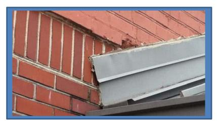
c. Remove and replace caulking at reglets, windows, and expansion/control joints.
